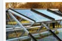
DOUBLE ROOF VENTS
